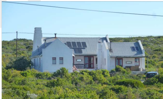
Rainwater tanks set under raised stoeps
