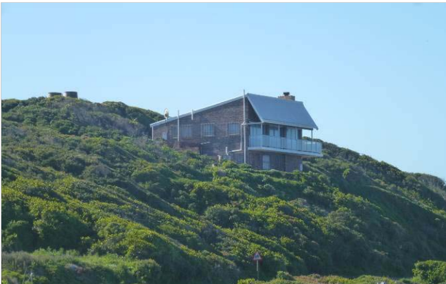
Impact of building protruding above skyline and with roof slope opposing contour gradient
