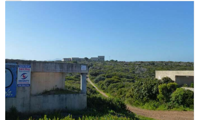
Gate and boundary wall on coastal drive
