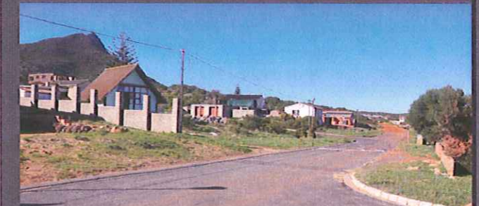
AREA 1 (Incomplete houses in west precinct)
