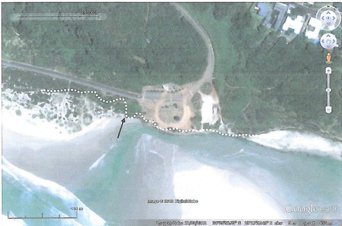
AERIAL PHOTO taken on 23 November 2012 showing the mouth breaching position opposite the Grotto parking area where the embankment of the parking area has been scoured away. Subsequent mouth breaching during the winter of 2013 has further back-eroded the fore dune in some areas to be only between 6-8 metres from the tar surface of the coastal tar road. The arrow indicates the position of the surface rocky outcrop that introduces further hydraulic phenomena that will further threaten the future of the coastal tar road.
