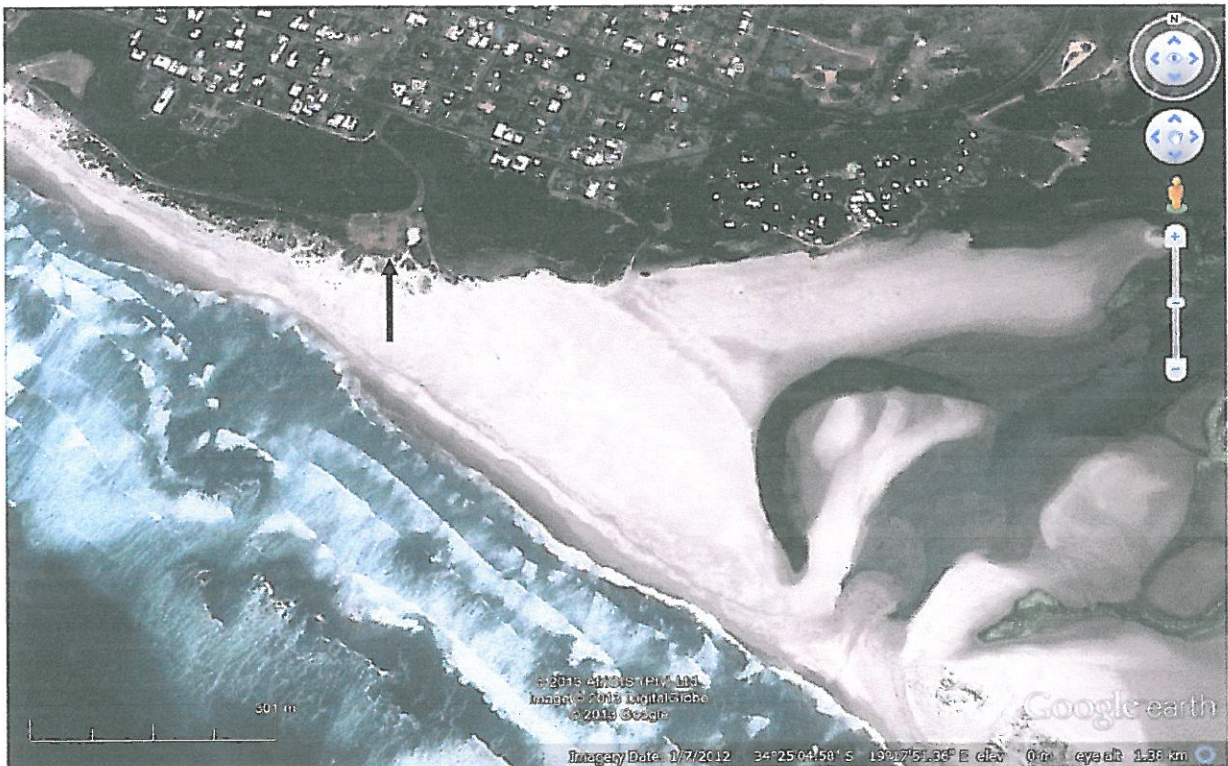
AERIAL PHOTO showing the location of the Grotto Bay parking area (marked with the arrow) where the protection works are to be implemented by means of some form of artificial stabilization of the bank of the parking area. Note the old area where the estuary breached that is now blocked by sand dunes from where sand will be sourced for the protection and to return the breach area further to the east of the parking lot.
