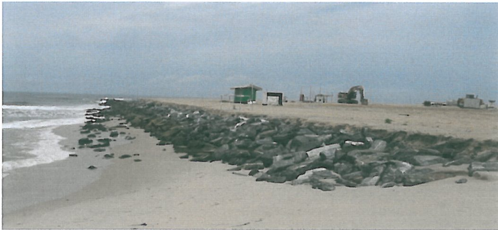
Figure 10: Rock protection Ghana
