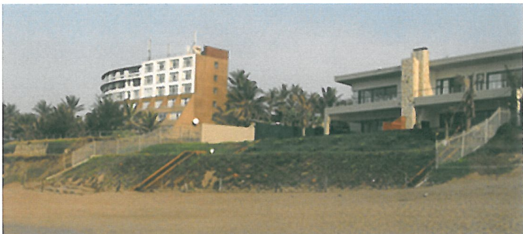
Figure 12: Shrimp Lane Ballito (note the vegetation on the sandbag slopes)
