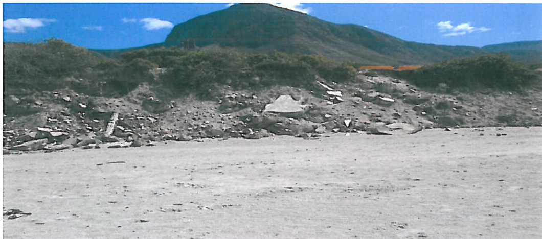
Figure 3: Eroded banks of the parking area (April 2013)
