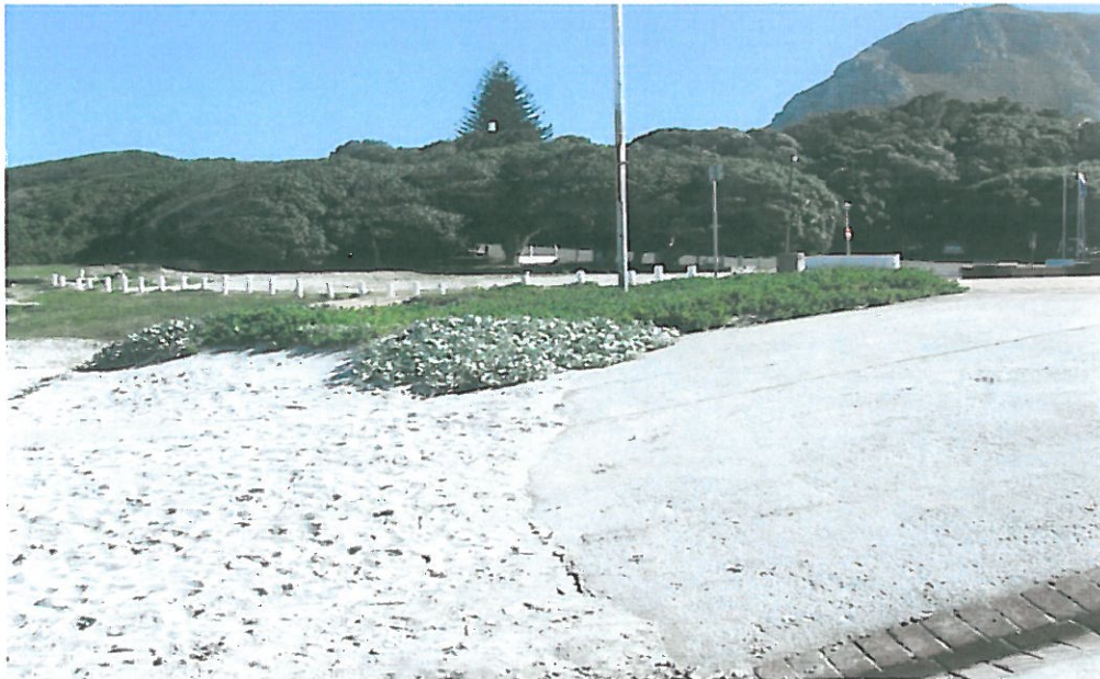
Figure 14: Concrete protection, Hermanus beach
